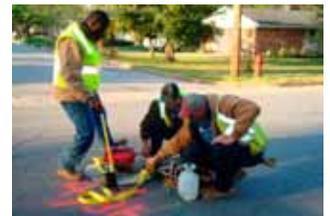
month. Line Maintenance personnel recently completed smoke testing on several quadrants of Perry's collection system with the support of Constantine Engineering. The results of this testing allowed the City of Perry to save more than \$1 million dollars in scheduled sewer upgrades.
